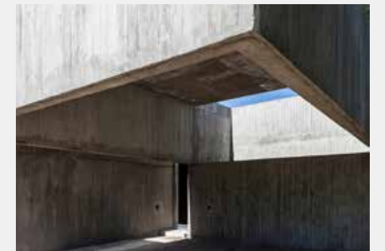
Close-up of concrete
