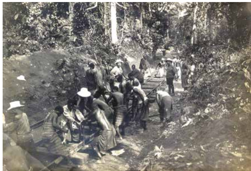
Congolese natives laying rails on the line of the Great Lakes Railway
