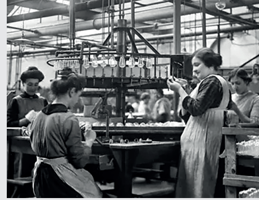
Workers at the factory.
