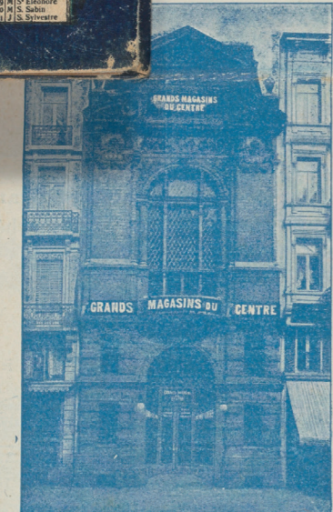
Facade principale. — 85, boulevard Anspach.
